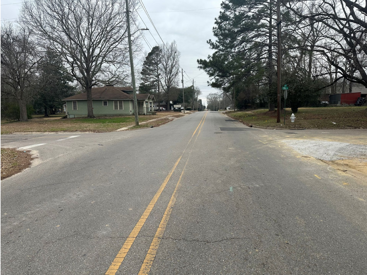
Figure 6.4: W 10 th Street east of N 11 th Avenue
